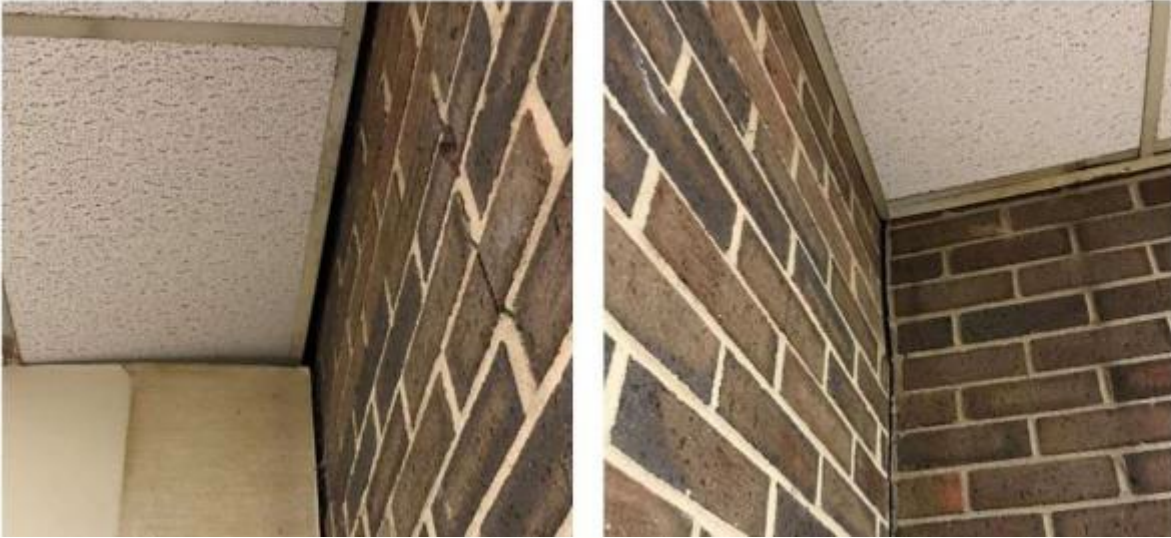
INTERIOR WALL DISPLACEMENT (POLICE)
