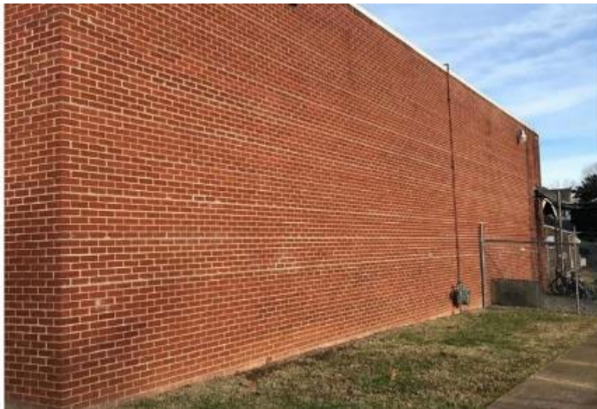
SOUTH WALL – PREVIOUS HORIZONTAL WALL CRACK REPAIR
