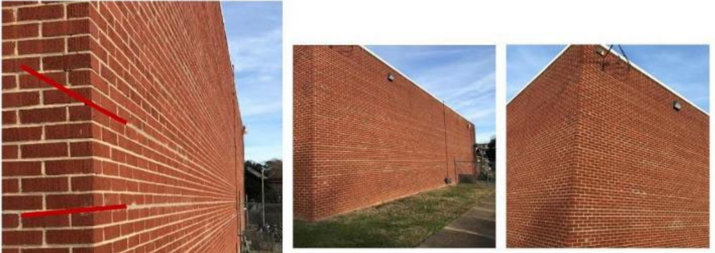
EXTERIOR HORIZONTAL WALL CRACK REPAIR
