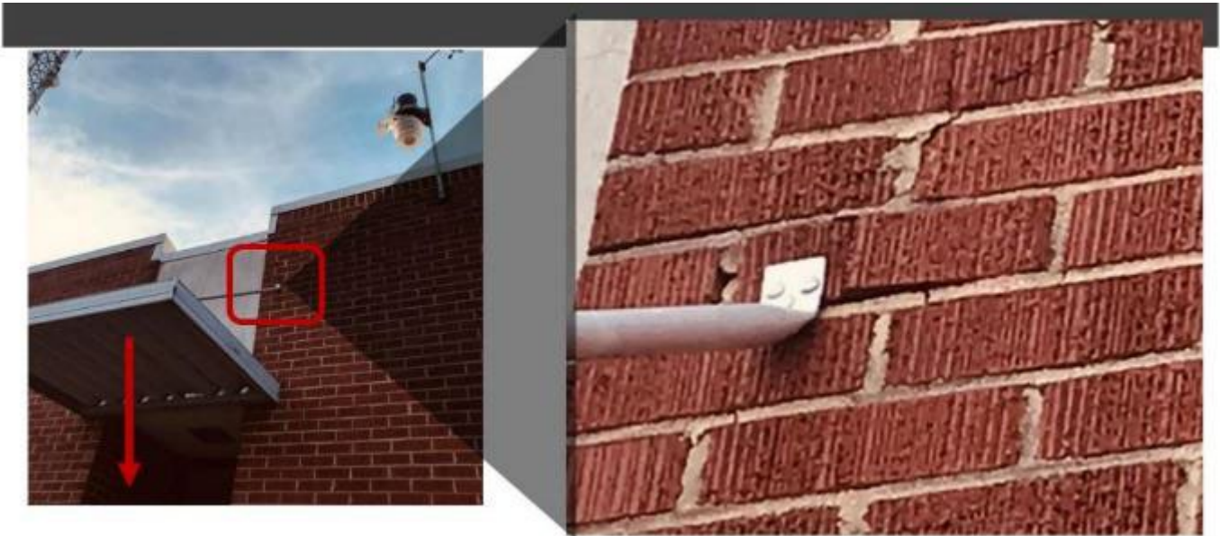
EAST WALL CANOPY / CRACKS
