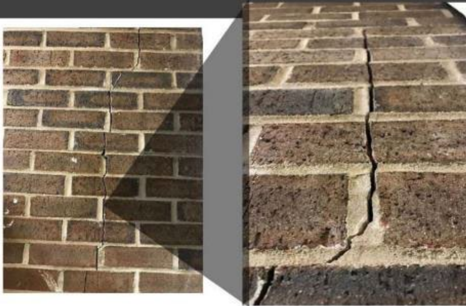
INTERIOR VERTICAL WALL CRACKS (POLICE)
