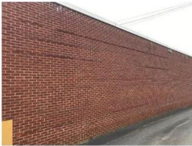
NORTH WALL CRACKS
