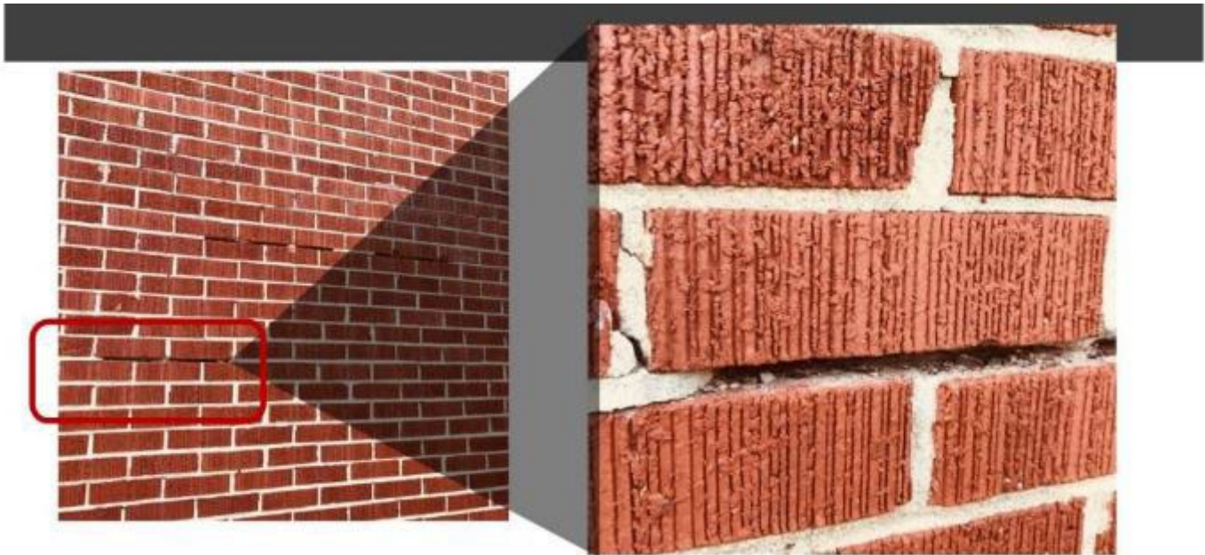
EAST WALL CRACKS
