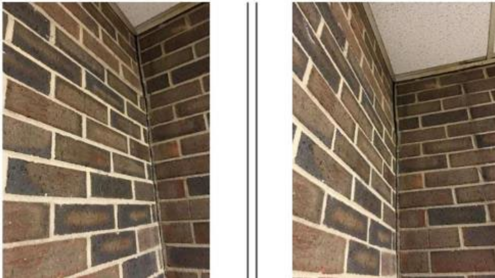
INTERIOR VERTICAL WALLS CRACKS (POLICE)
