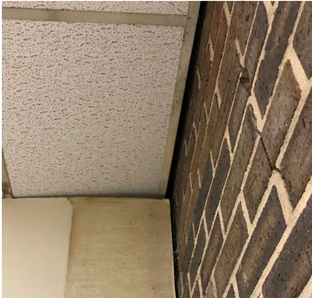
Interior Wall Displacement (Police)
