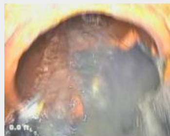
Bottom Right Portion of Pipe is Missing
