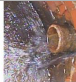
MH 2712 Severe Leak (View from MH)
