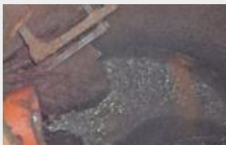
MH 1634 Heavy Roots in Pipe Seal & Active Leak
