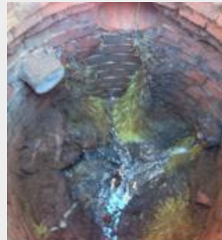
MH 1266 Large Penetration of Roots & Mud, Steady Infiltration Under SL
