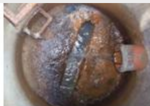
MH 1383 Joint Leaks
