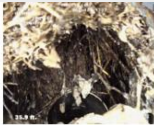
Tap Is Partially Missing, Cavity Exists Above Main & SL, Active Infiltration, Flow Exiting Out, Roots, Heavy Debris Buildup
