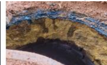
MH 1660 Deteriorated Frame
