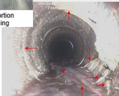
Tap Break-In Caused Multiple Breaks in Pipe
