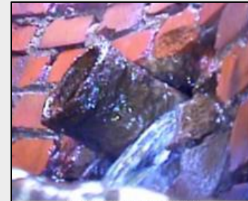
MH 2712 Severe Leak (View from CCTV camera)
