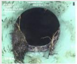
Defective PVC/Truss Connection with Roots & Gaps
