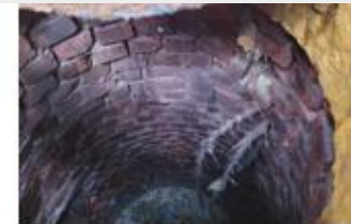
MH 1660 Large Roots & Missing Bricks
