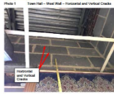
Vertical cracks in mortar joints and through middle of block.
