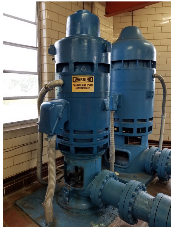
Water Treatment Plant Motor Control Centers – High Service Pump Replacement
