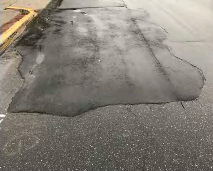
Asphalt Patch for Water Line Repair in Main Street
