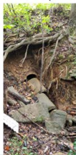
Erosion undercutting Pineburr(North side)
