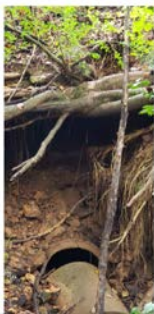
Erosion undercutting Pineburr(North side)
