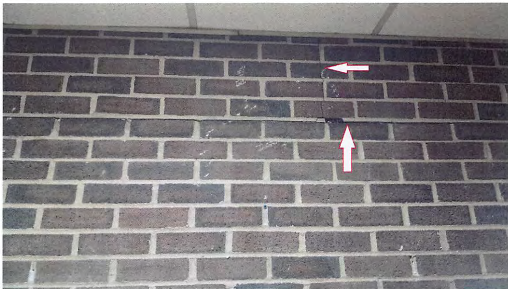
ANOTHER VIEW OF THE SAME CRACK IN SQUAD ROOM SHOWING VERTICAL PORTION OF CRACK.
