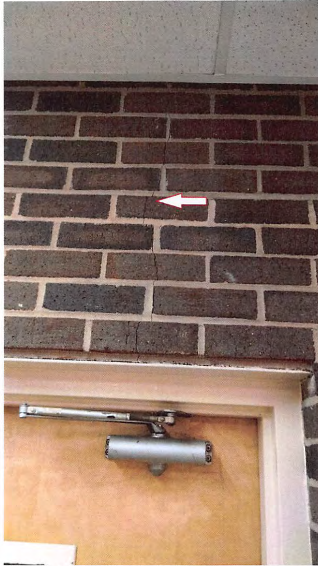
VERTICAL CRACK ABOVE DOOR NEAR FIRE CHIEF'S OFFICE.
