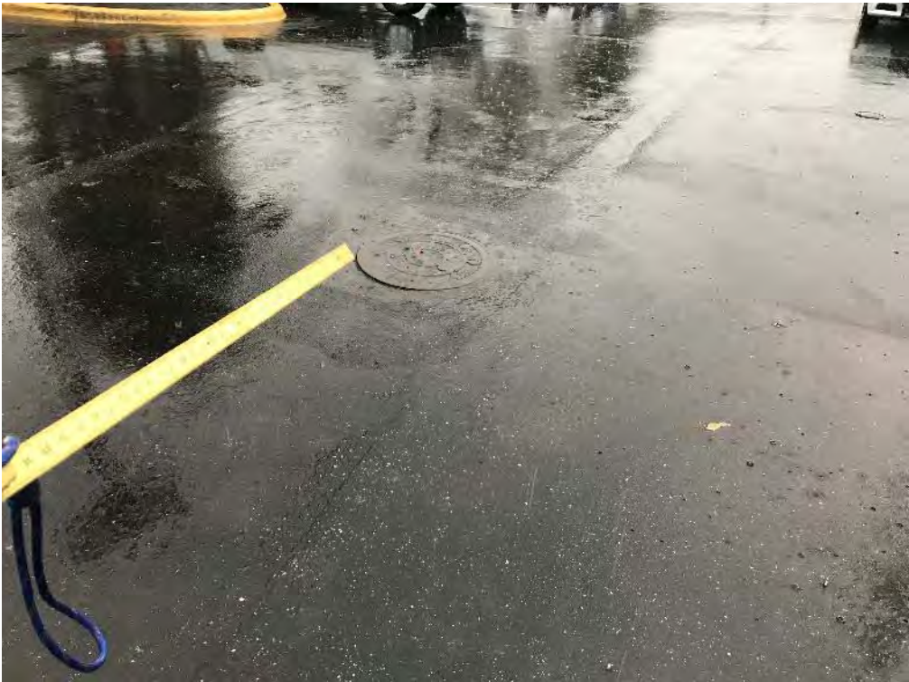
Photo 19 Public Safety Building – East Side – Manhole
