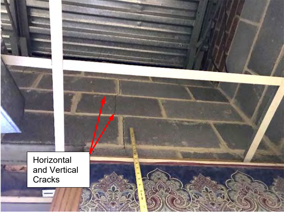
Photo 2 Town Hall – West Wall – Horizontal and Vertical Cracks
