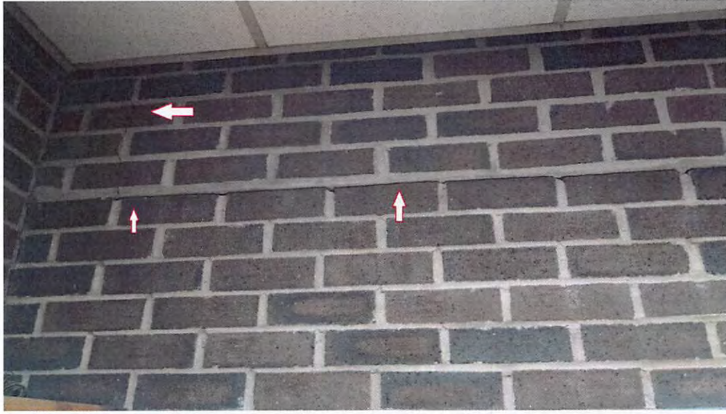
VIEW OF A DIFFERENT HORIZONTAL AND VERTICAL CRACK IN WALL OF ARMS ROOM.
