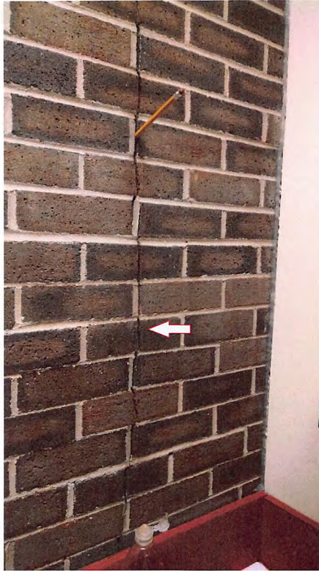
ANOTHER VIEW OF THE CRACK IN THE FINGERPRINTING ROOM WALL. THIS CRACK EXTENDS FROM THE FLOOR TO THE CEILING.
