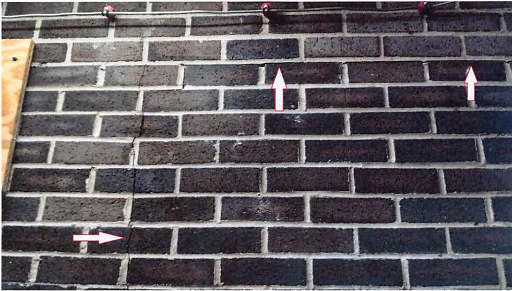
HORIZONTAL AND VERTICAL CRACK IN WALL IN SERVER ROOM.
