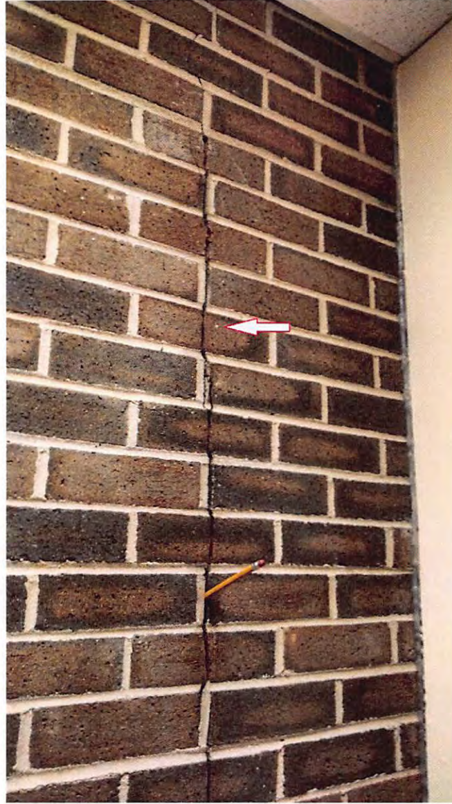
VERTICAL CRACK IN FINGERPRINTING ROOM WALL. THIS WALL IS AN EXTERIOR WALL.
