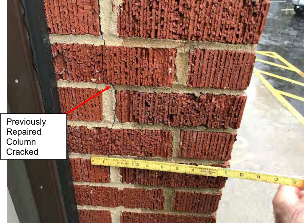
Photo 22 Public Safety Building – East Side – Cracked Column
