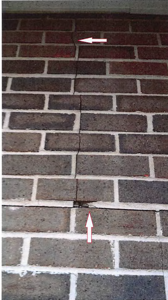
VERTICAL AND HORIZONTAL CRACKS IN WALL OF FIRE CHIEF'S OFFICE. VERTICAL CRACK EXTENDS FROM FLOOR TO CEILING. THIS WALL IS AN EXTERIOR WALL.
