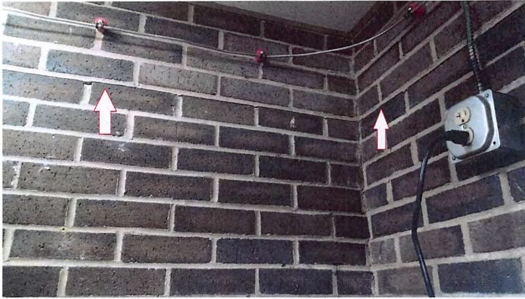
HORIZONTAL CRACK ALONG WALL IN SERVER ROOM.
