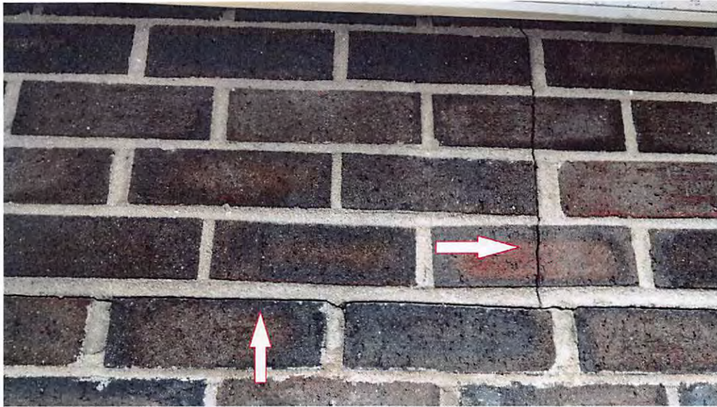
VERTICAL AND HORIZONTAL CRACK IN INTERVIEW ROOM WALL.
