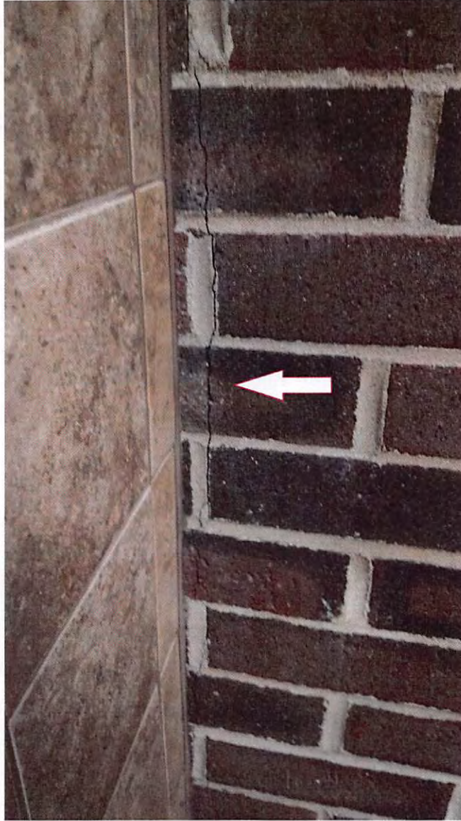
VERTICAL CRACK IN WALL IN MEN'S RESTROOM. THIS IS AN INTERIOR WALL.
