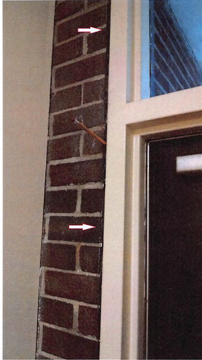
ANOTHER VIEW OF WALL SEPARATING FROM DOOR FRAME ON EXTERIOR DOOR ON EAST SIDE OF BUILDING.
