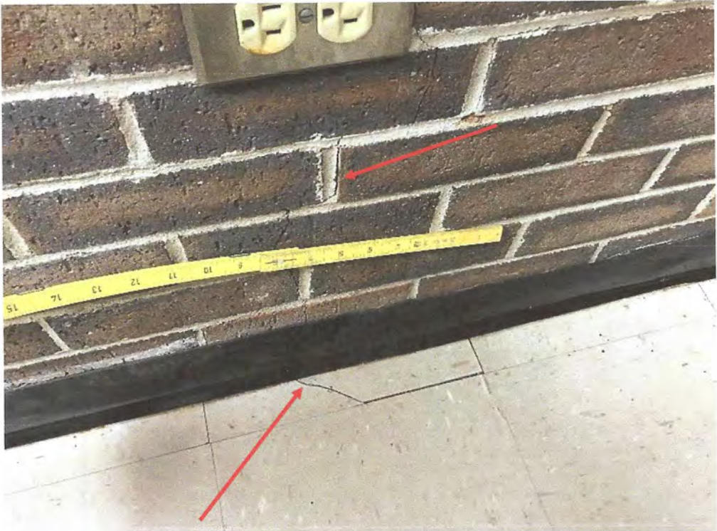
Photo 28 Public Safety Building – West Wall – Wall and Slab Crack
