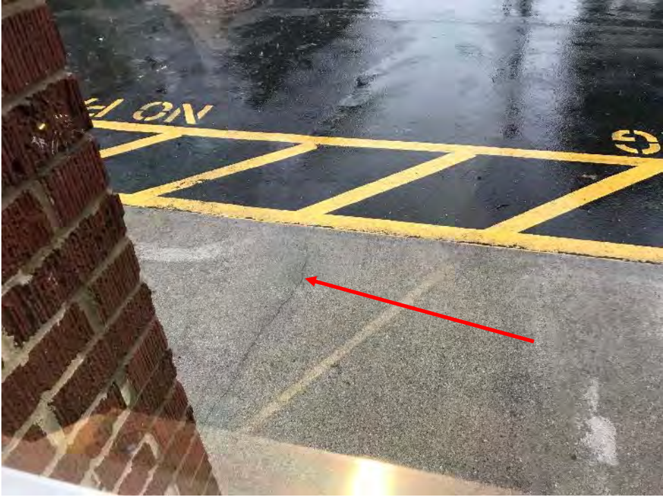
Photo 21 Public Safety Building – East Side – Cracked Slab
