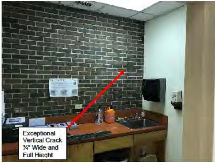
Photo 10 Public Safety Building – East Wall – Vertical Crack
