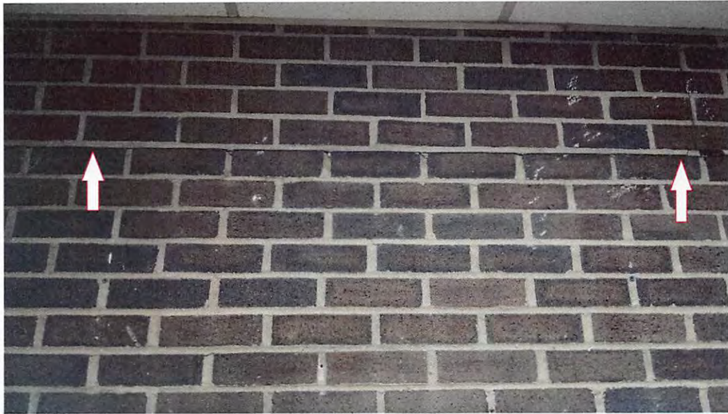
VIEW OF ANOTHER HORIZONTAL AND VERTICAL CRACK IN SQUAD ROOM.
