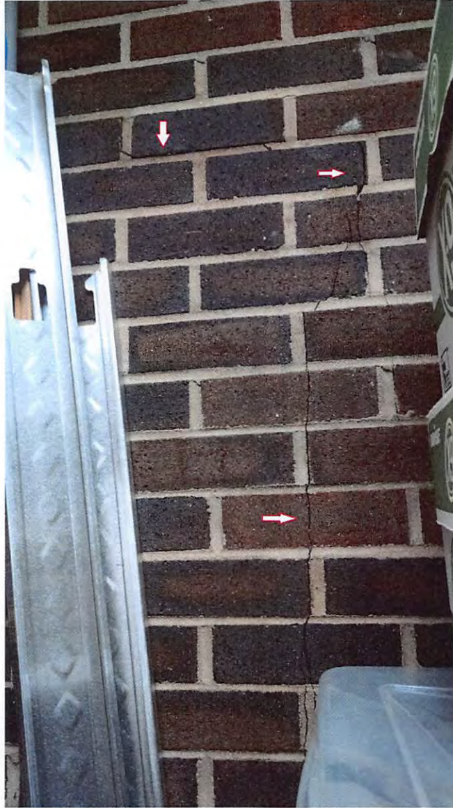
HORIZONTAL AND VERTICAL CRACK IN WALL IN ARMS ROOM.
