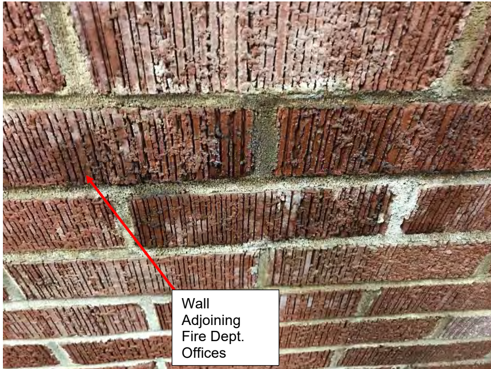
Photo 23 Public Safety Building – Engine Bay – Efflorescence
