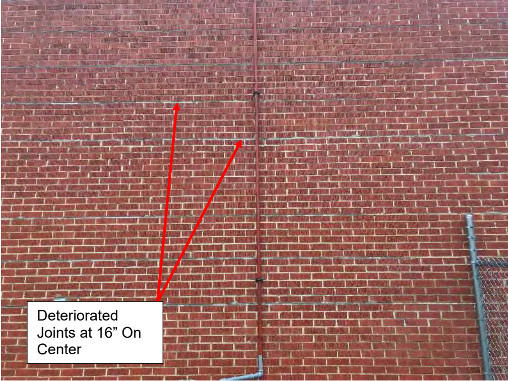
Photo 15 Public Safety Building – South Wall – Deteriorated Joints
