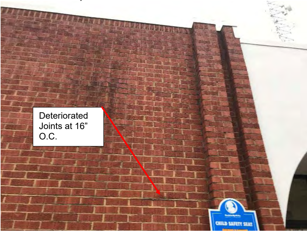
Photo 18 Public Safety Building – West Wall – Deteriorated Joints
