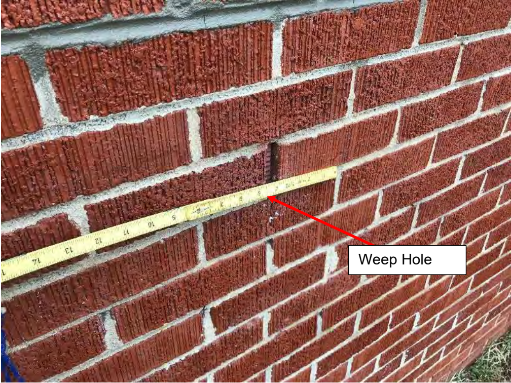
Photo 17 Public Safety Building – South Wall – Repaired Joint and Weep
