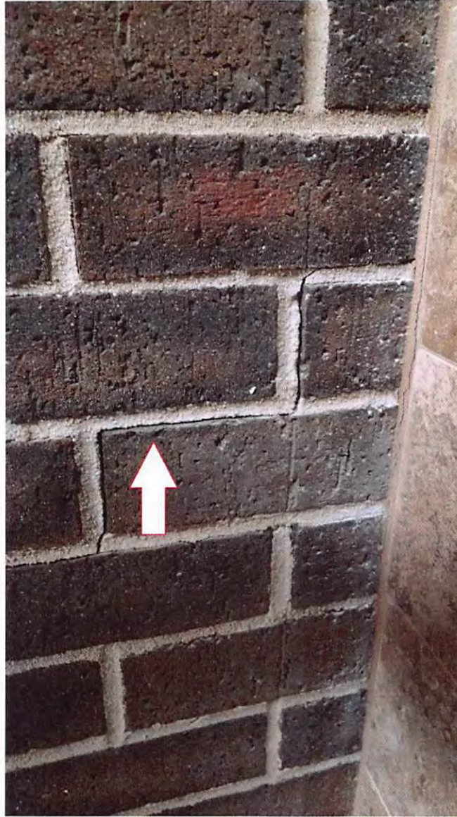
VERTICAL AND HORIZONTAL CRACK IN WALL OF WOMEN'S REST ROOM.
