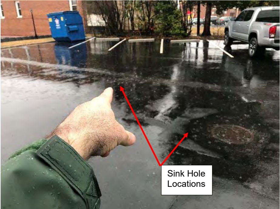
Photo 20 Public Safety Building – East Side – Historical Sink Hole
