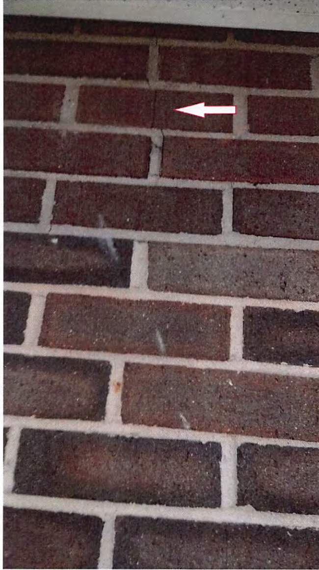
VERTICAL AND HORIZONTAL CRACKS IN INTERVIEW ROOM WALL. THIS WALL IS AN EXTERIOR WALL.
