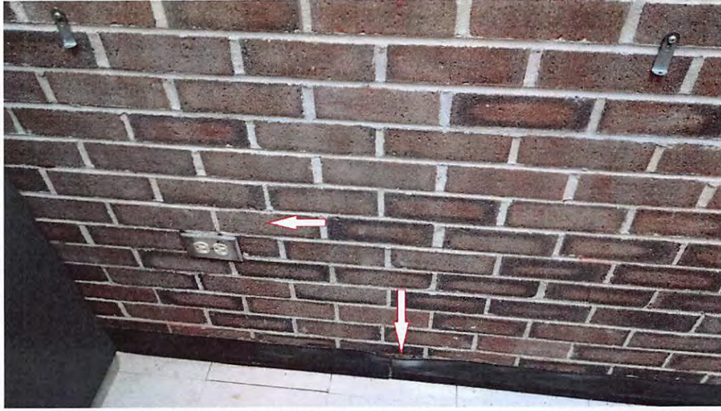
VIEW OF ANOTHER CRACK IN WALL OF POLICE CHIEF'S OFFICE. FLOOR IS SEPARATING FROM WALL. THIS IS AN EXTERIOR WALL.
