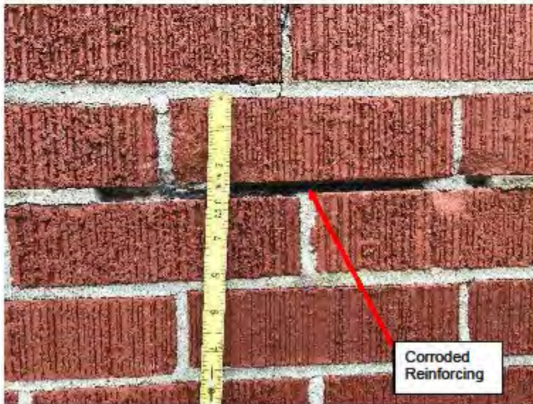
Photo 16 Public Safety Building – South Wall – Deteriorated Joints
