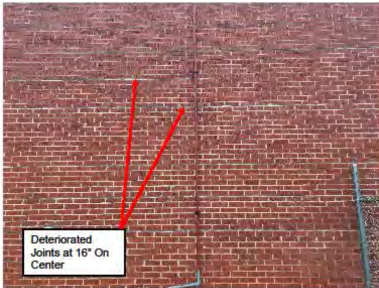
Photo 15 Public Safety Building – South Wall – Deteriorated Joints
