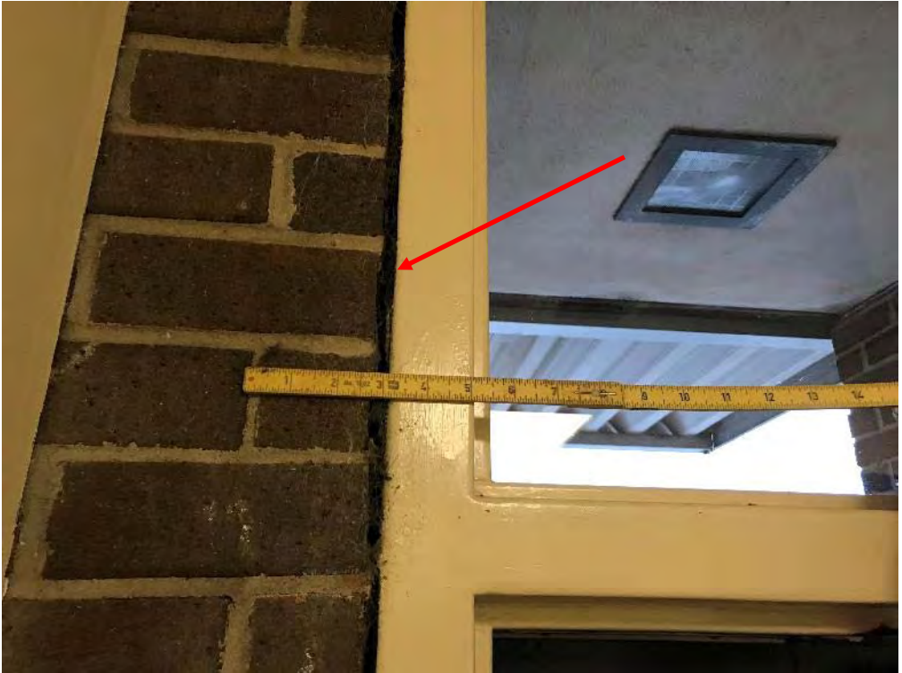
Photo 26 Public Safety Building – East Wall – Separation at Door Frame
