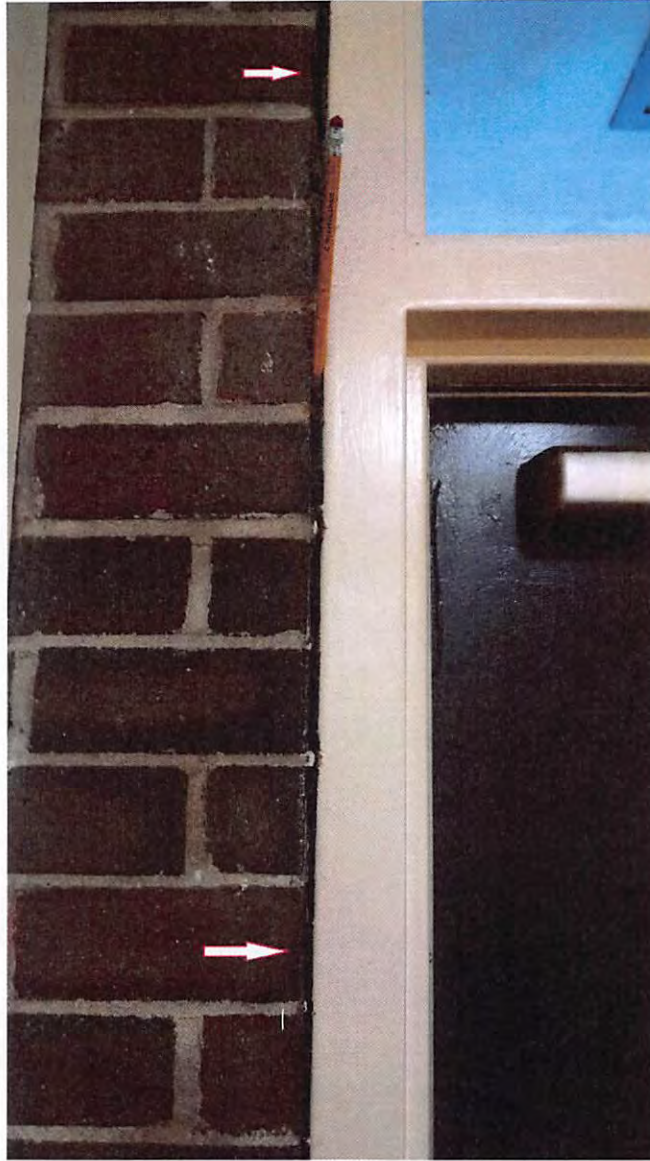
WALL SEPARATING FROM DOOR FRAME ON EXTERIOR DOOR ON EAST SIDE OF BUILDING. THIS IS AN EXTERIOR WALL.
