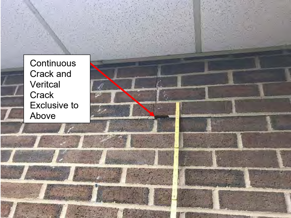
Photo 13 Public Safety Building – South Wall – Horizontal Crack
