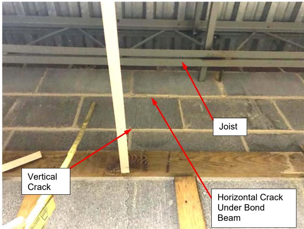
Photo 3 Town Hall – South Wall – Horizontal and Vertical Cracks
