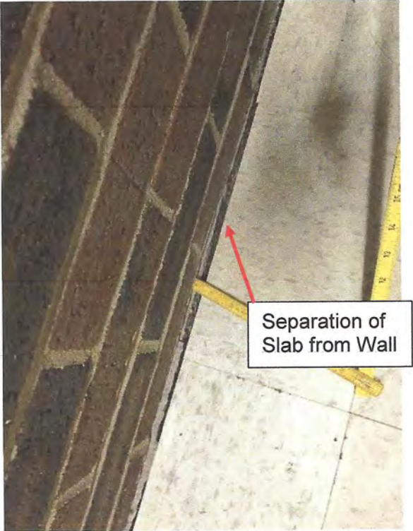
Photo 27 Public Safety Building – East Wall IT Room – Wall Separation
