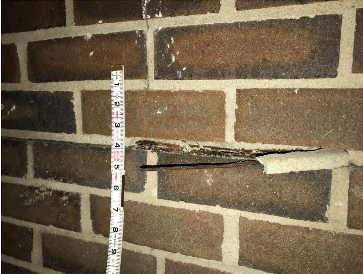
Photo 2 – 100% corroded wire reinforcing (examples were discovered in both Chief Watts office and the room adjacent to Chief Moss's office in December 2018)
