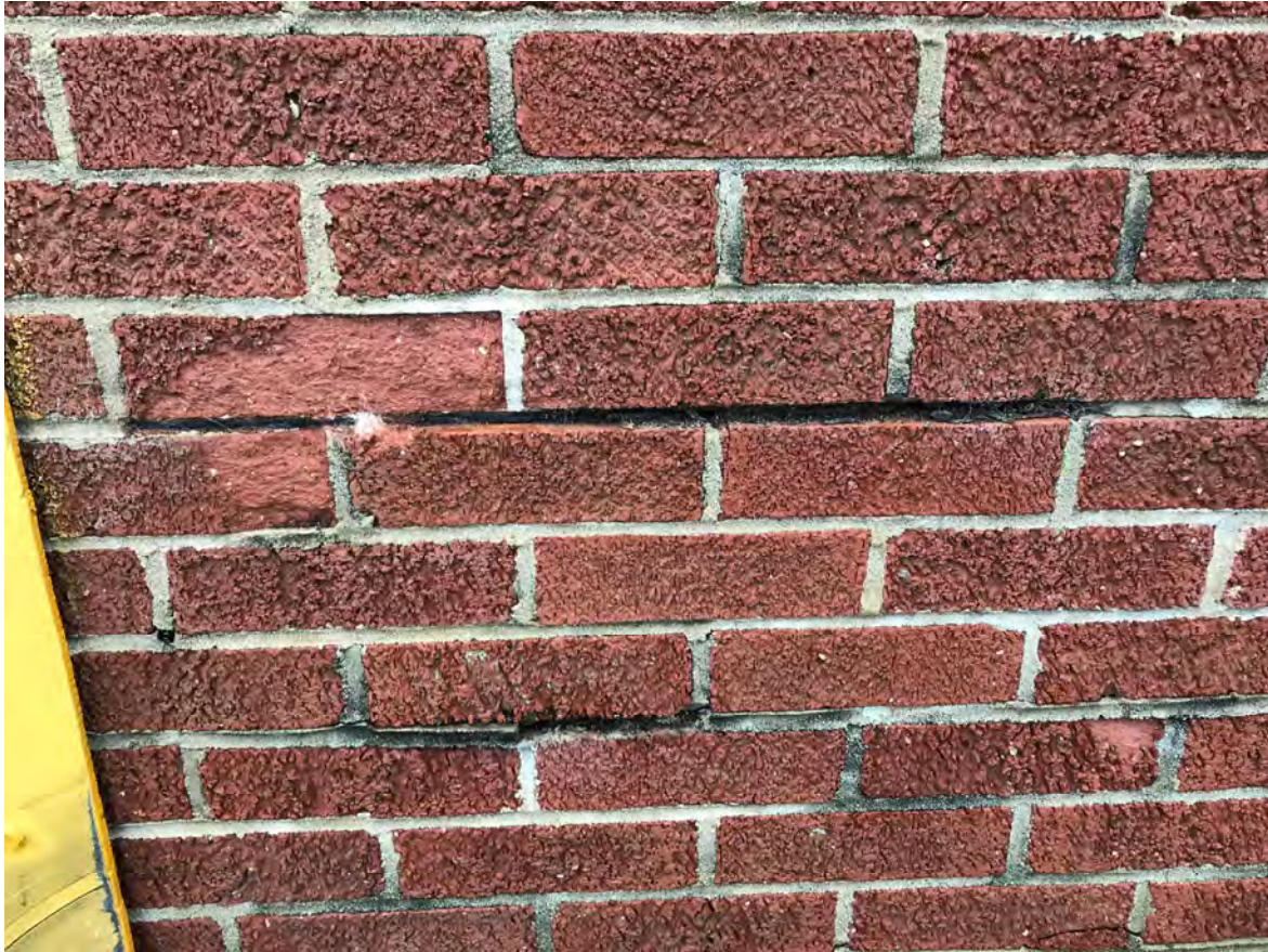
Photo 1 – Exterior Brick with Obvious Severe and often 100% Reinforcing Corrosion and Mortar Spalling
