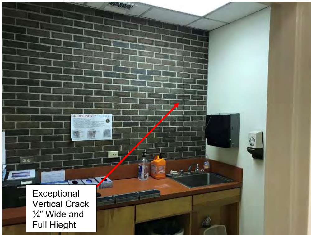
Photo 10 Public Safety Building – East Wall – Vertical Crack
