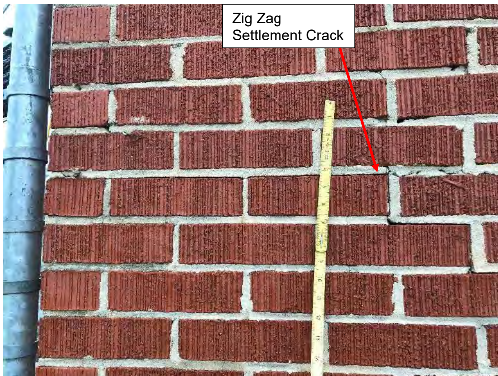
Photo 14 Public Safety Building – Southeast Corner – Zig Zag Crack
