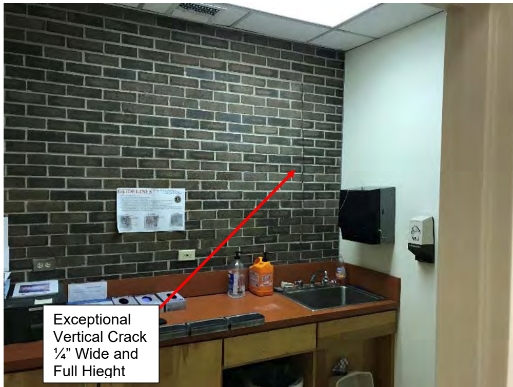
Photo 10 Public Safety Building – East Wall –Vertical Crack
