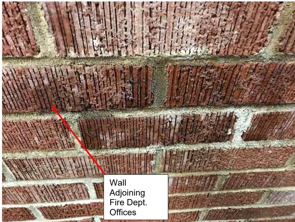
Photo 23 Public Safety Building – Engine Bay – Efflorescence
