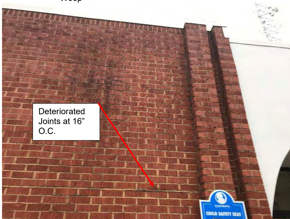
Photo 18 Public Safety Building – West Wall – Deteriorated Joints
