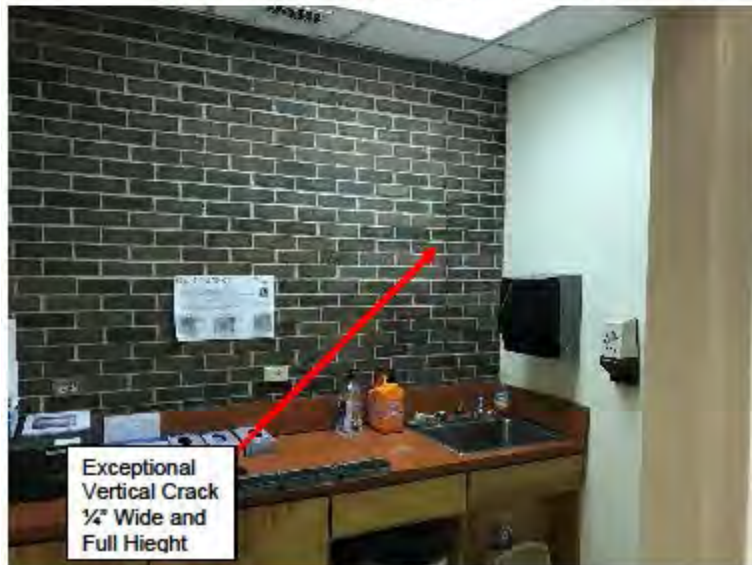
Photo 10 Public Safety Building – East Wall – Vertical Crack
