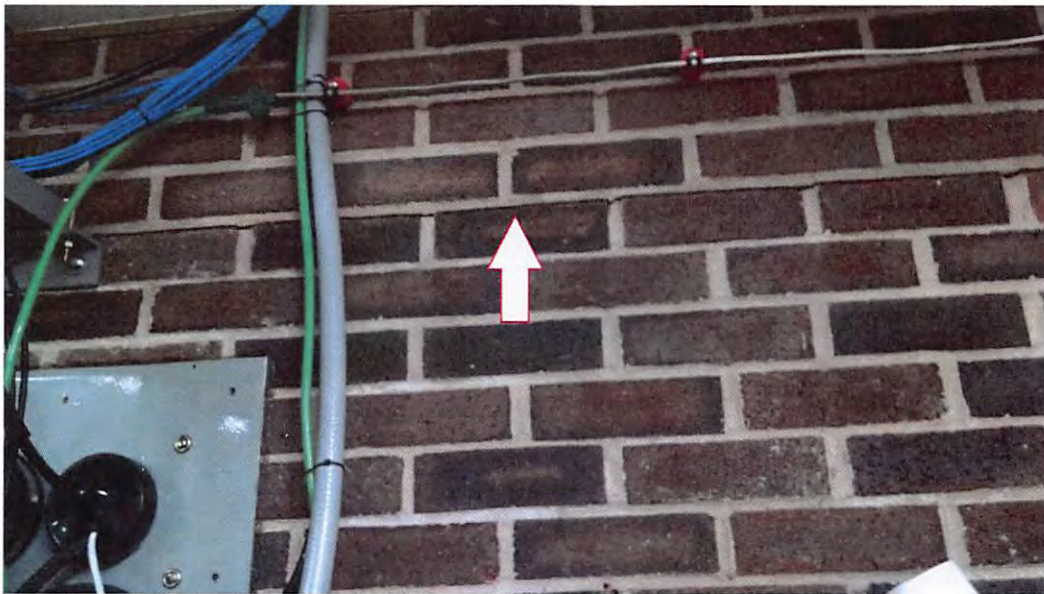
HORIZONTAL CRACK ALONG WALL IN SERVER ROOM.
