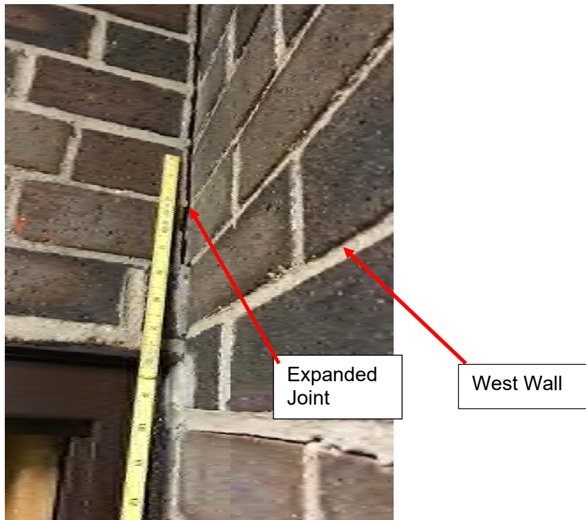
Photo 8 Public Safety Building – West Wall – Expanded Joint/Crack
