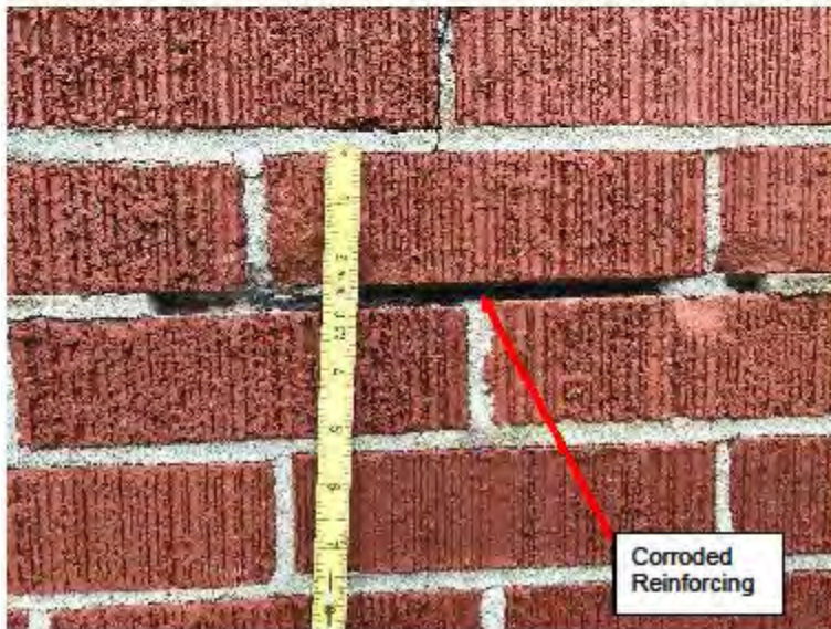
Photo 16 Public Safety Building – South Wall – Deteriorated Joints
