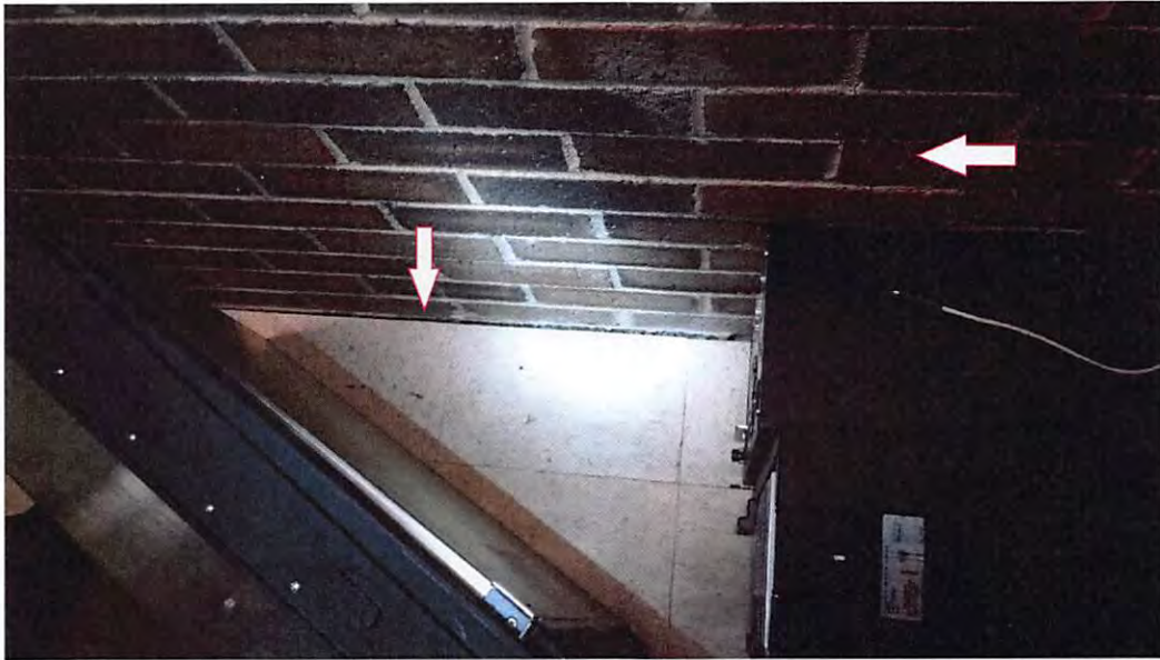
HORIZONTAL AND VERTICAL CRACK IN WALL IN SERVER ROOM. FLOOR HAS ALSO SUNKEN AND MOVED AWAY FROM WALL.
