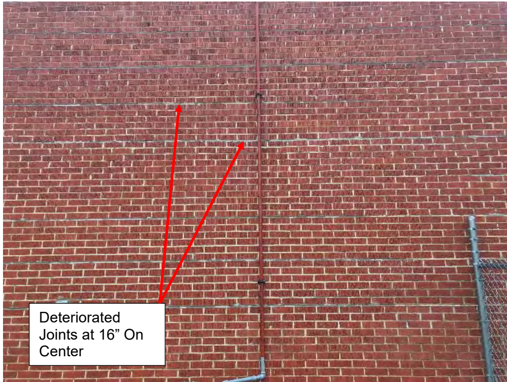
Photo 15 Public Safety Building – South Wall – Deteriorated Joints
