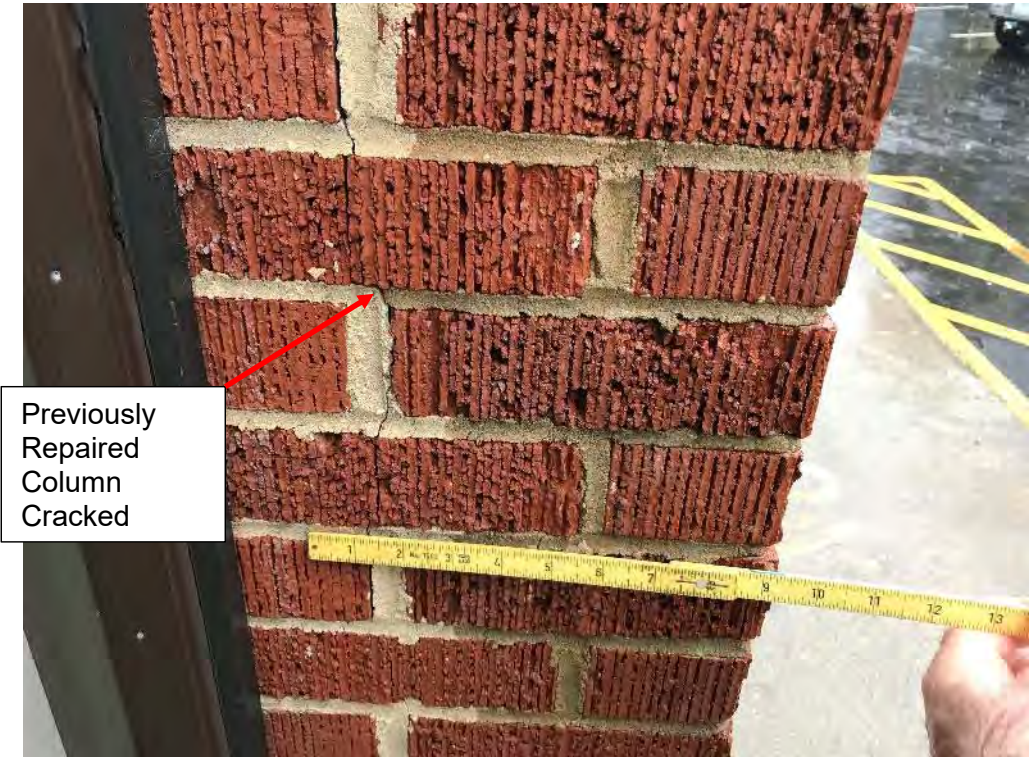
Photo 22 Public Safety Building – East Side – Cracked Column
