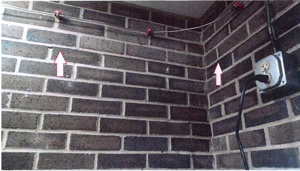
HORIZONTAL CRACK ALONG WALL IN SERVER ROOM.
