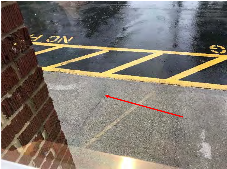
Photo 21 Public Safety Building – East Side – Cracked Slab
