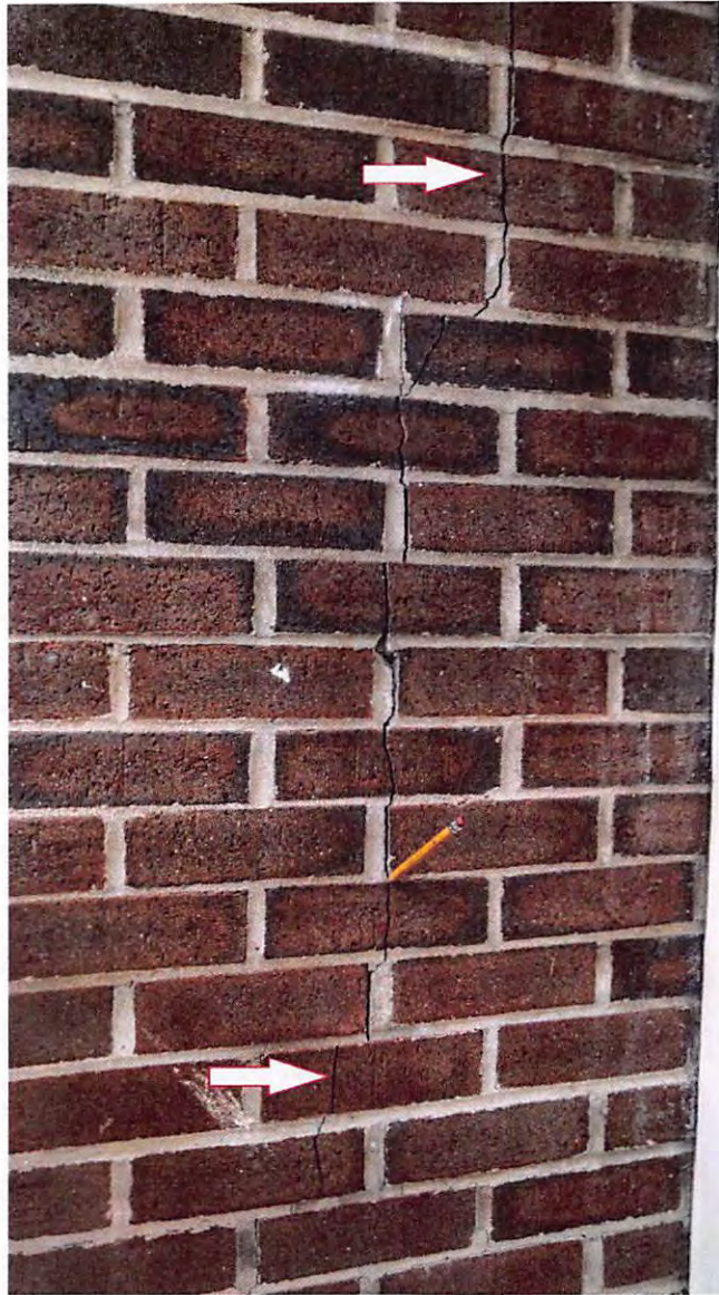
VERTICAL CRACK IN WALL IN WALL IN SQUAD ROOM. THIS IS AN EXTERIOR WALL.
