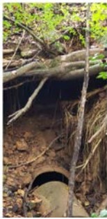
Erosion undercutting Pineburr(North side)
