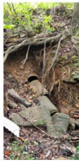
Erosion undercutting Pineburr(North side)
