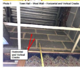
Vertical cracks in mortar joints and through middle of block.
