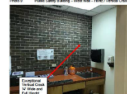
Some vertical cracks run full height of wall on interior of building.
