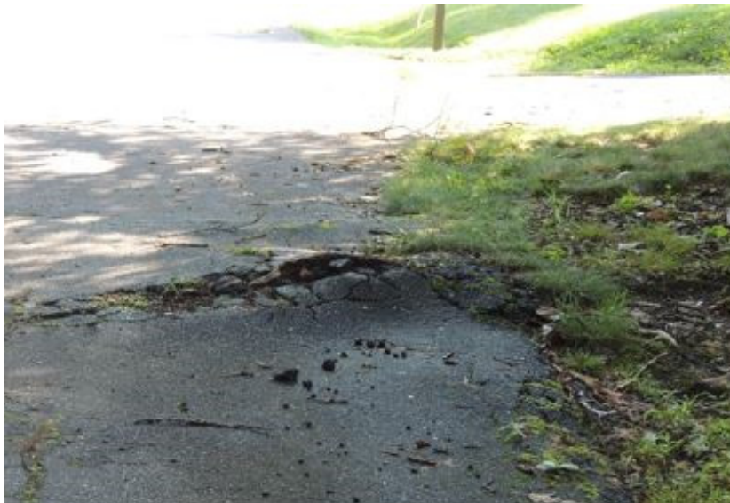
Figure 5 Root Damage
