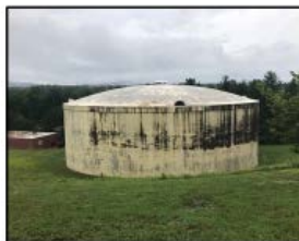
Water Treatment Plant – Finished Water Clearwell
