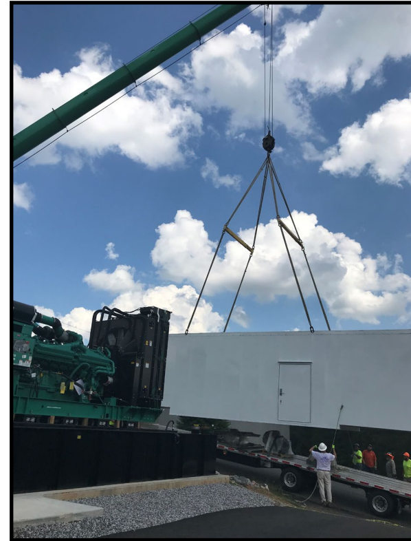
Water Treatment Plant – Backup Generator
