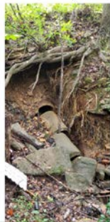
Erosion undercutting Pineburr(North side)
