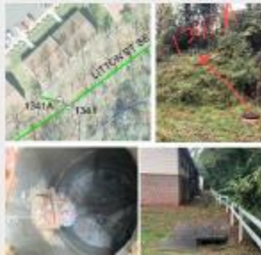
UNRESOLVED ISSUE (POSSIBLE STORM PIPE CONNECTION)
