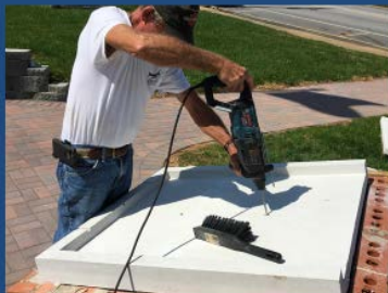
Document Tray Being Placed and Secured DOCUMENT TRAY BEING PLACED ON TOP OF FOUNDATION SUPER-STRUCTURE
