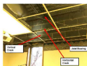
Old Town Hall Wing of Building Cracks in load bearing masonry block walls.
